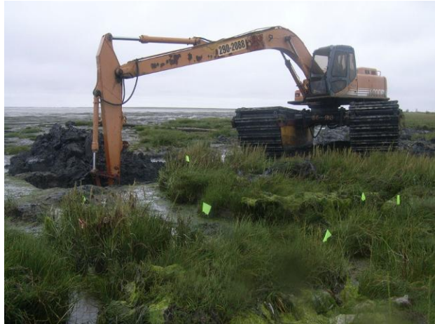
Figure 12. Linkbelt Excavator Removing S. anglica at Brunswick Point, BC - 2010.
