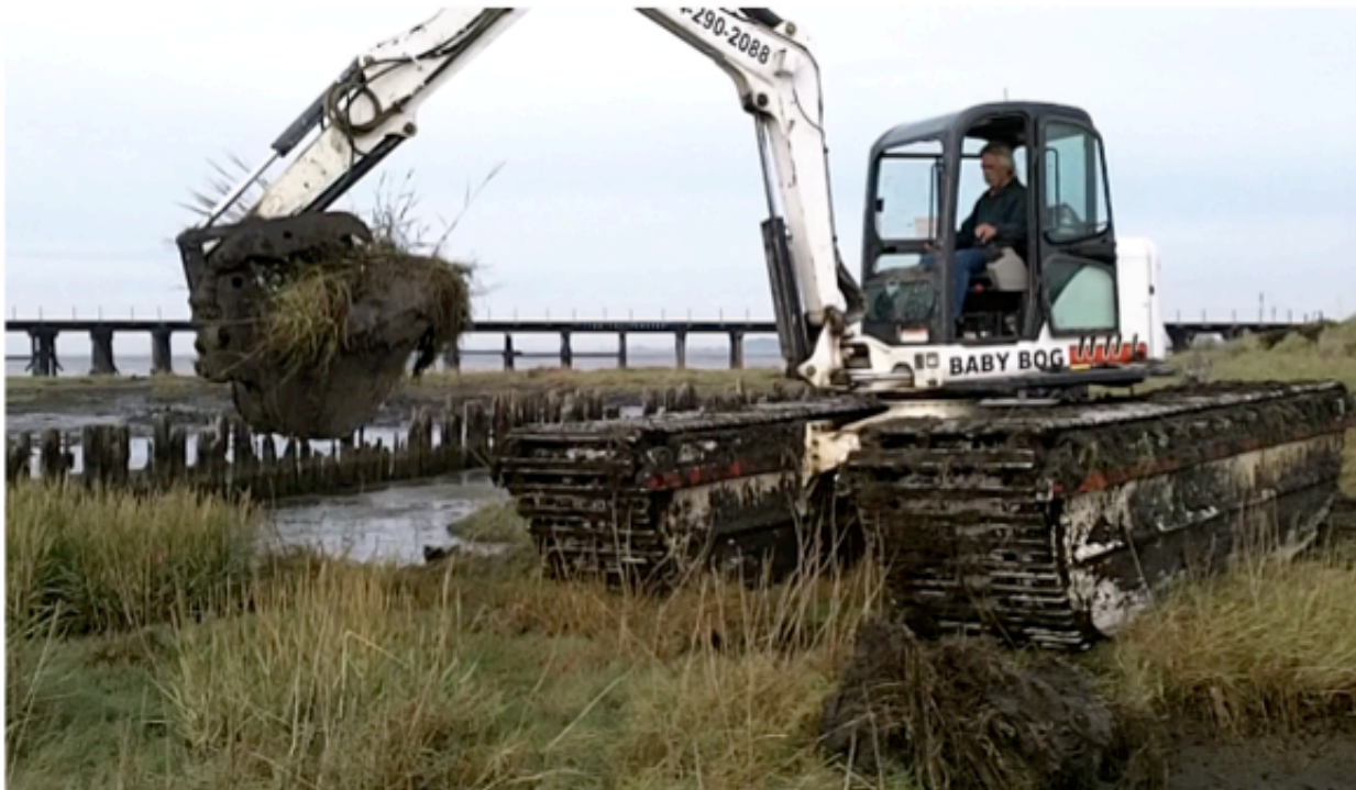
Figure 15. Amphibious Excavator Removing S. anglica , Mud Bay, 2012
